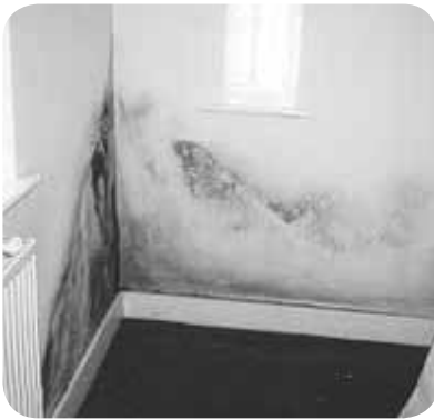
▲ Walls with black mould growth
