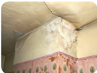
▲ Internal penetrating damp
